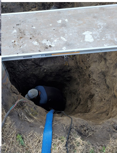
Photo left: the joys of high iron, hard groundwater. Photos to right: digging out the pitless adaptor and having to pump out the water due to the high water table.
